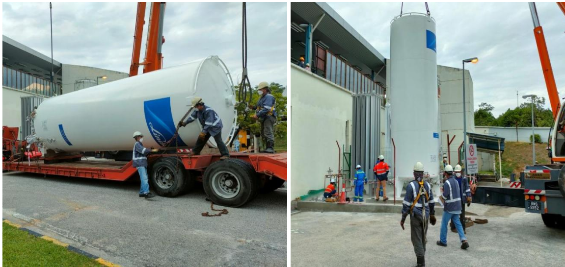
Gambar rajah 1: Pemasangan tangki VIE di Hospital Sungai Buloh
