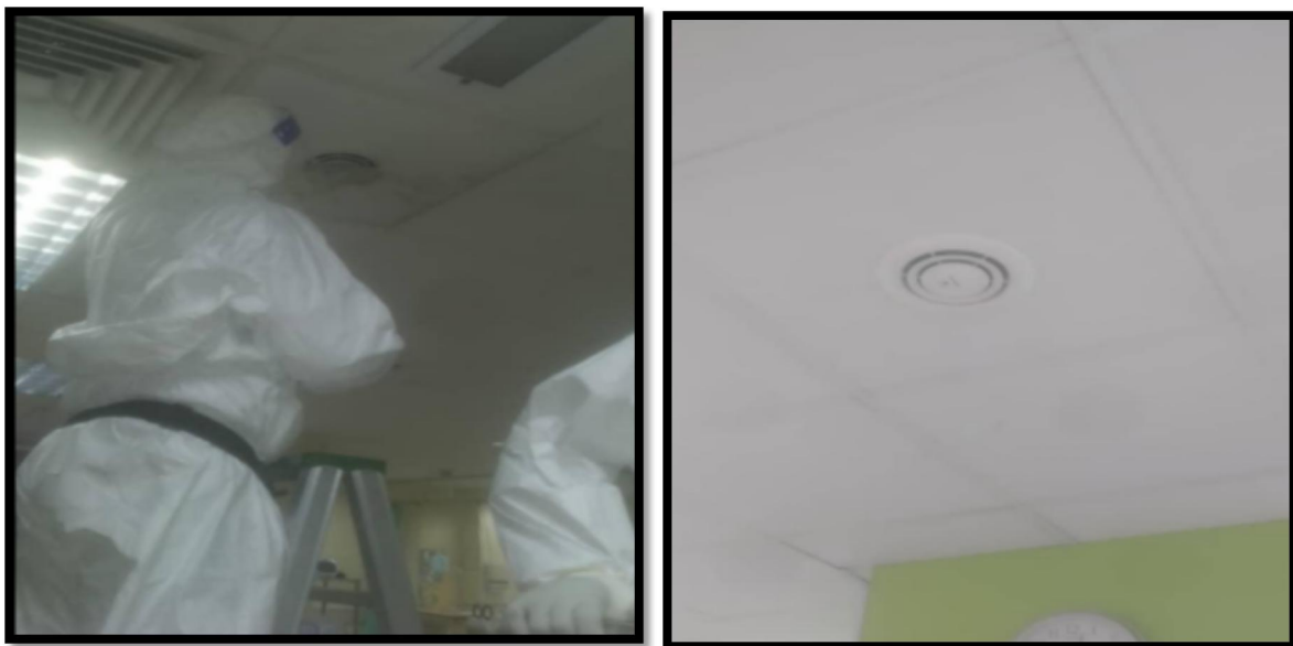
Gambar rajah 5: Pemasangan Nano-E di Hospital Sungai Buloh
