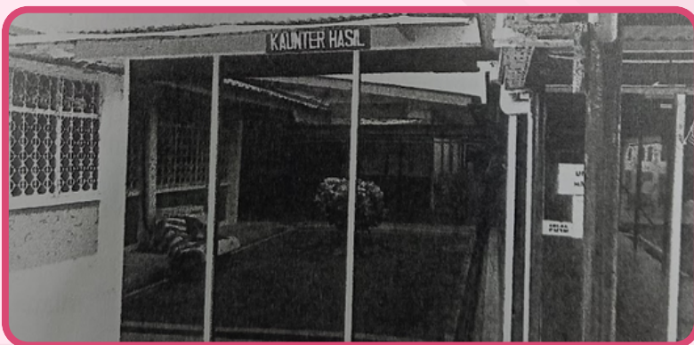
Tinted cermin selesai dipasang
